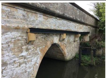
**FIGURE 10 – GENERAL VIEW OF STEEL JOIST AND STONE CORBEL**
