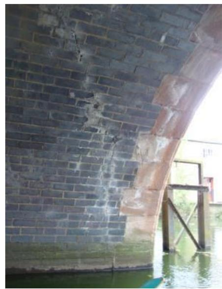
**FIGURE 3 - CIRCUMFERENTIAL CRACKING WITH LEACHING**
