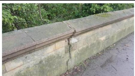
**FIGURE 9 – CRACKING AND TWISTING OF PARAPET WALL**
