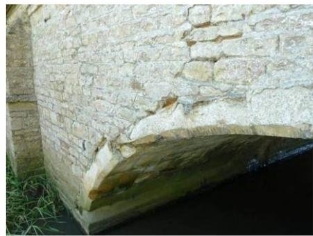
**FIGURE 8 – CRACKING AND DAMAGED STONWORK**
